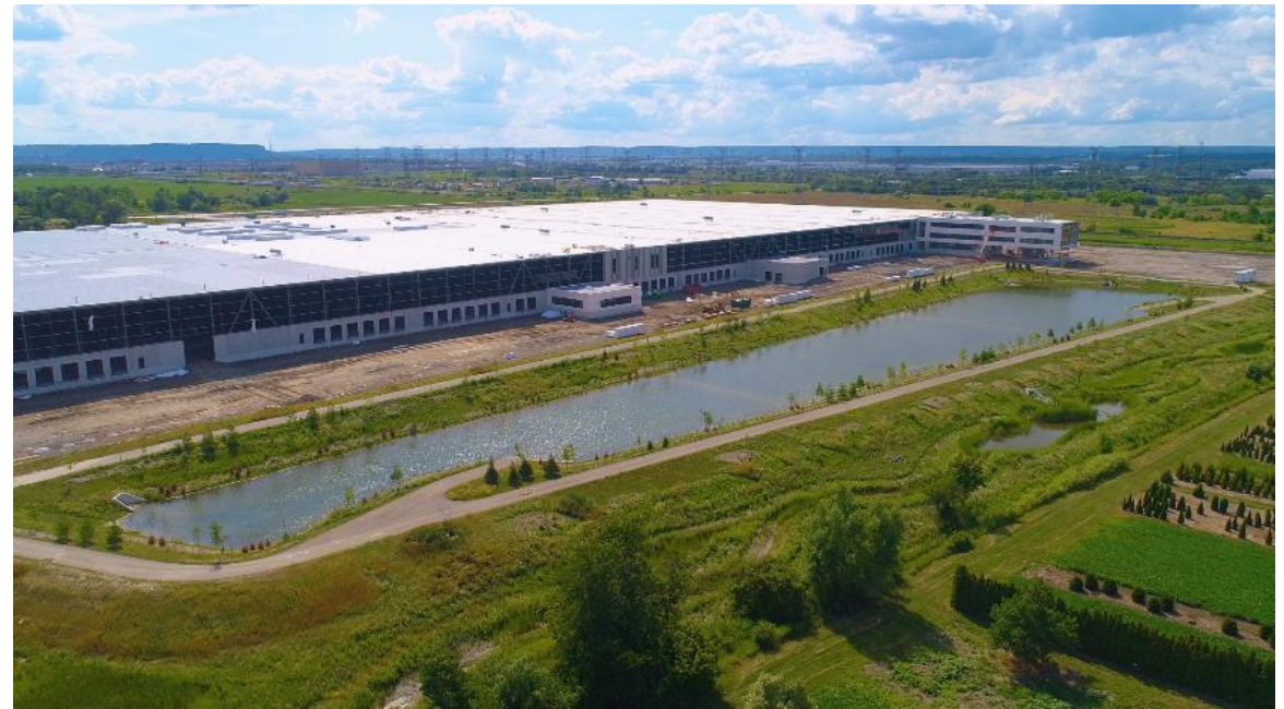
DSV's Milton logistics facility – 1.2 million sq. ft, opened Feb 2020
