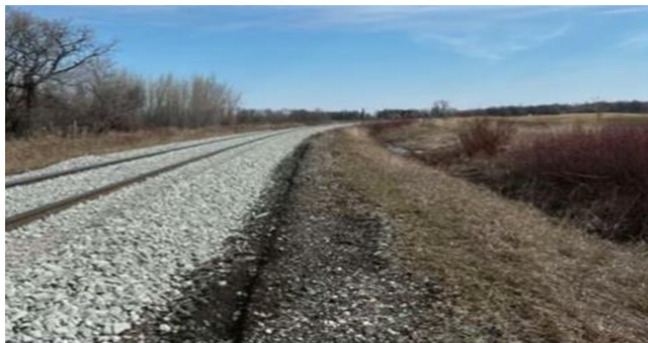
North of Emerson MP 61.6 after track lift (May 4)
