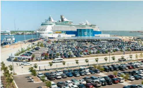
An internal roadway and on-site parking at Cruise Terminal 10 help reduce traffic congestion and speed up passenger boarding.
